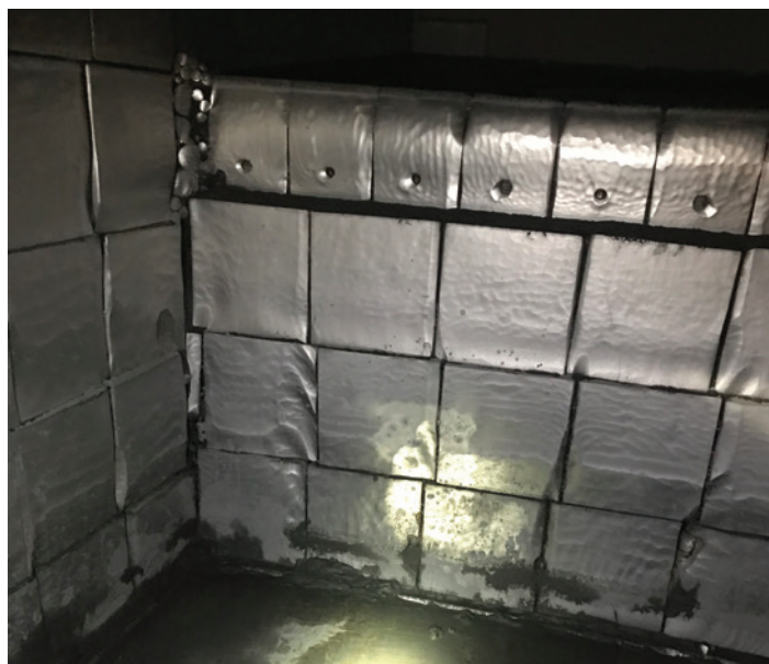
Ni-Hard liners installed in a pump box
